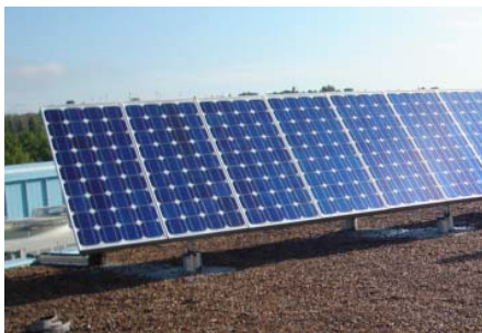
Figure 2. Front of a roof-mounted PV array
