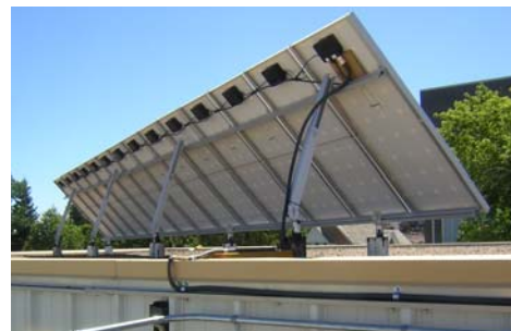
Figure 3. Rear of a roof-mounted PV array
